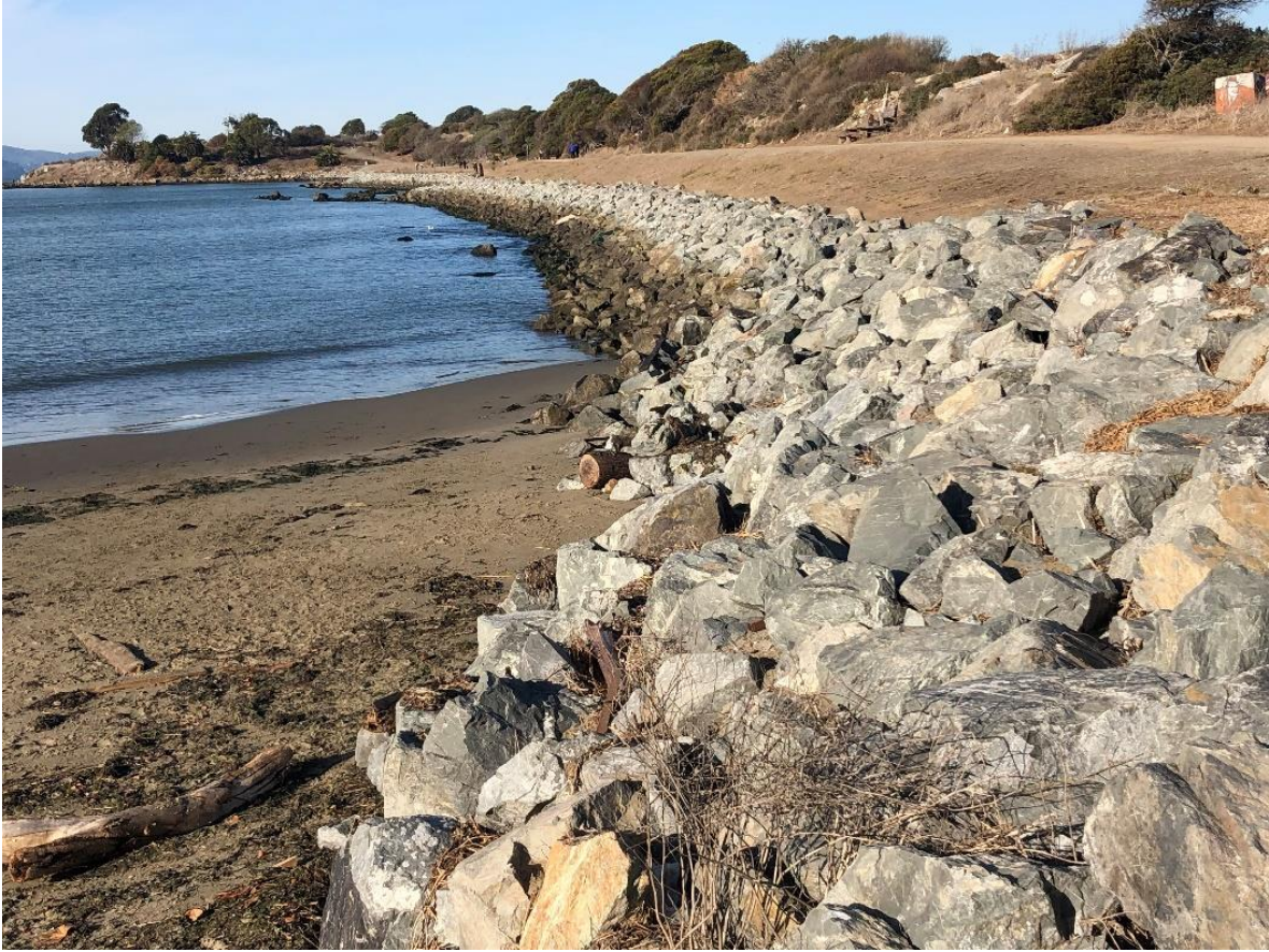
Figure 13 Armored Rock Revetment at Albany Shore
