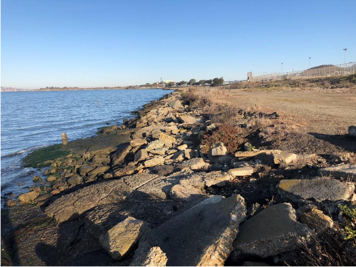
Figure 14 Filled Reclaimed Areas with Rubble at North Basin Strip, McLaughlin Eastshore State Park
